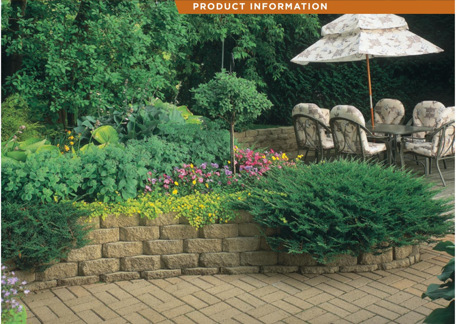
The traditional face style of the Windsor Stone<sup>®</sup> retaining wall system gives any garden wall a timeless appearance. Lightweight and easy to handle, the Windsor Stone block is the perfect choice for projects up to 2 feet high, including the buried course, but excluding the cap.\* A matching cap completes the system.
