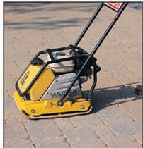
3. Pass the plate compactor\* over the entire surface to compact the sand.
