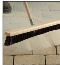
6. Remove excess sand from the surface with the broom.
