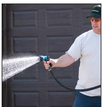
9. Starting from bottom of the slope, quickly shower a 200 sq. ft. section to set the sand. Immediately afterwards, wet the same section for **30 seconds**.
