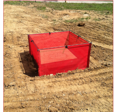
"Big Red" AI Protector, recently installed with trenched in bottom and tight sides.
