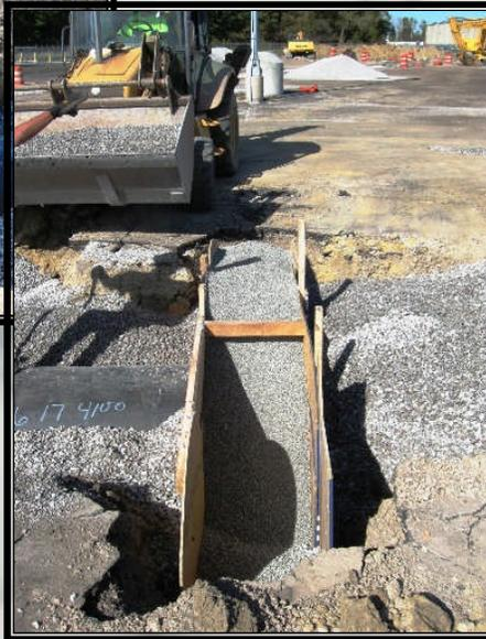
When placed in a trench perpendicular to a sewer line or other conduit (as pictured at left), product can be wetted to produce a durable, structurally stable barrier that maintains a very low permeability. The coating of individual particles swells against the exterior sidewalls of the pipe and “self-keys” into surrounding soil without the need for benching, installation in lifts, or manual re-compaction. The result: an economical and technically superior barrier.
