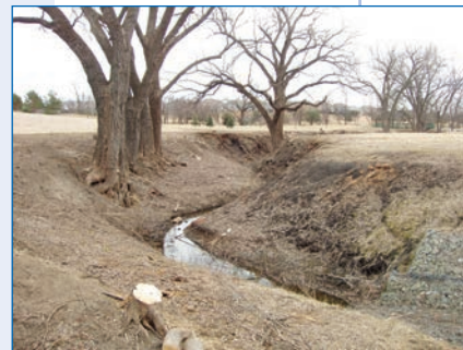
2 Channel before installation.
