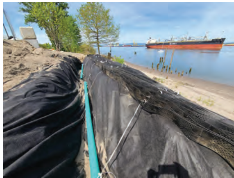
After River Walk Installation w/ Presto Geoweb Support
