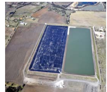
Waste Water Treatment Plant
