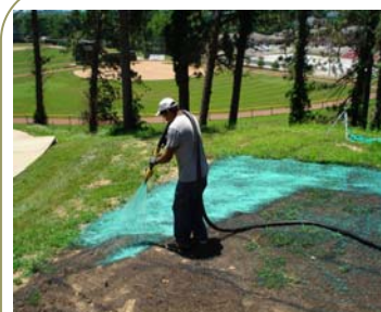
Hydraulically applying Flexterra FGM in and on the Enkamat TRM structure
