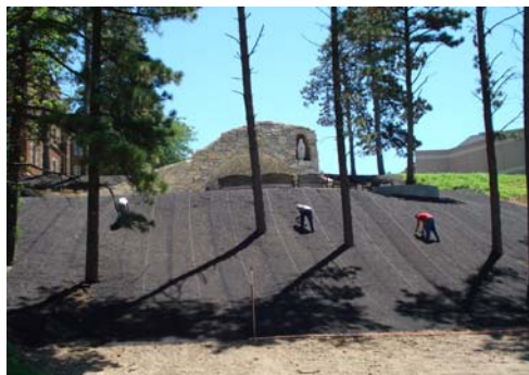
Installing the Enkamat base.
