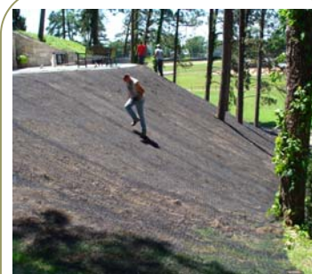
3 dimensional TRM Structure installed with 6" staples
